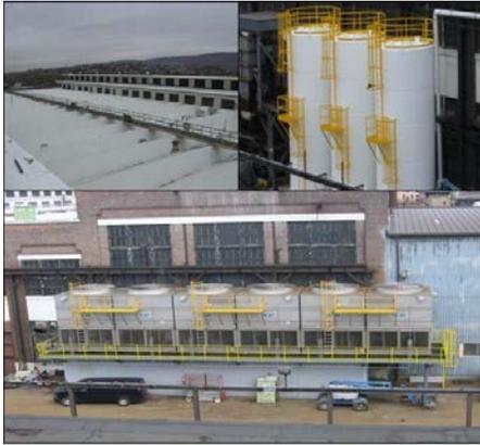
**Photo 5: Array of SCAAP Rainwater Collection System.**
